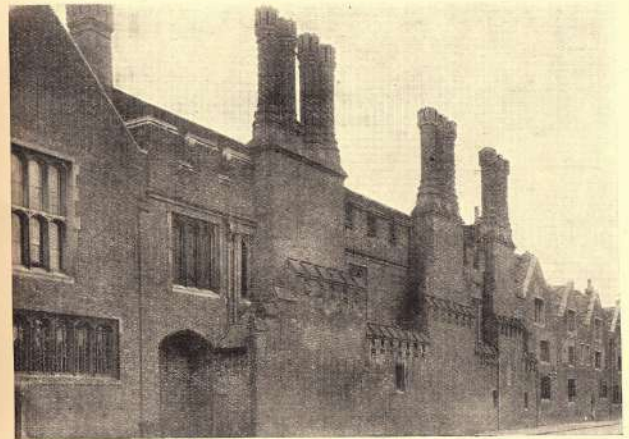
CHIMNEYS OF THE KING'S GREAT KITCHEN
